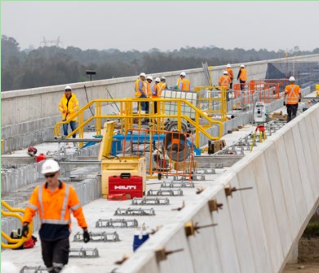
Sydney Metro construction between Orchard Hills and Luddenham
